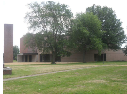
Charger Community Center, 2010
